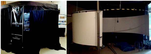
Figure 6. A.R.T.E. structure: exterior and interior view.
